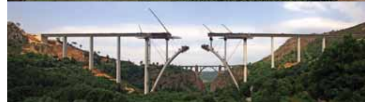
1. Viaduct of the Ulla river
