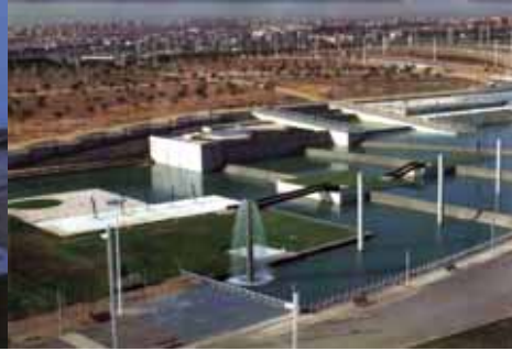
5. Design and construction of the Artificial Lake Juan Carlos I Park. Madrid
