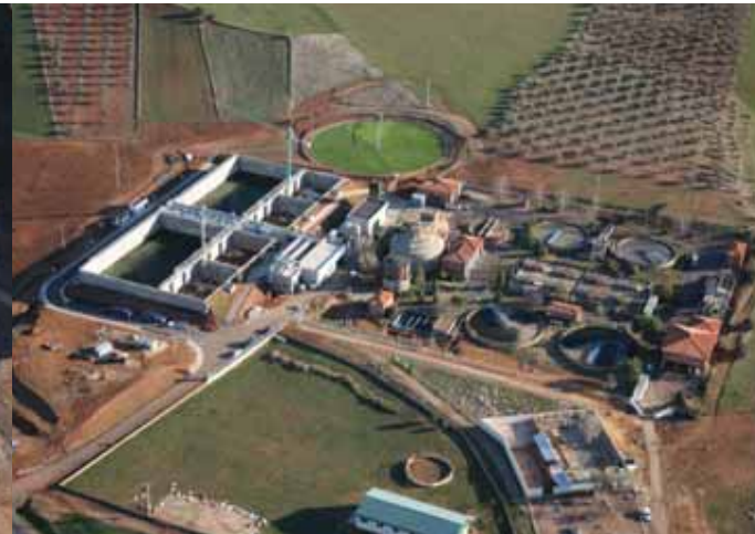
4. Design and construction supervision of the Puertollano wastewater treatment infrastructure
