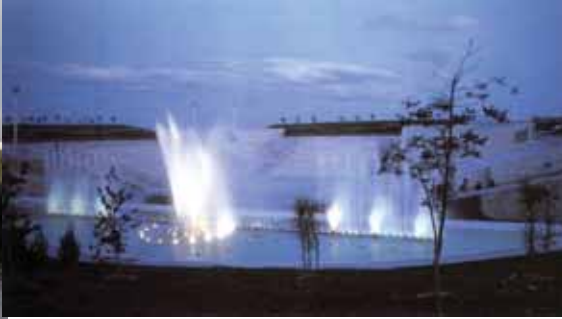
4. Design and construction of the Artificial Lake Juan Carlos I Park. Madrid
