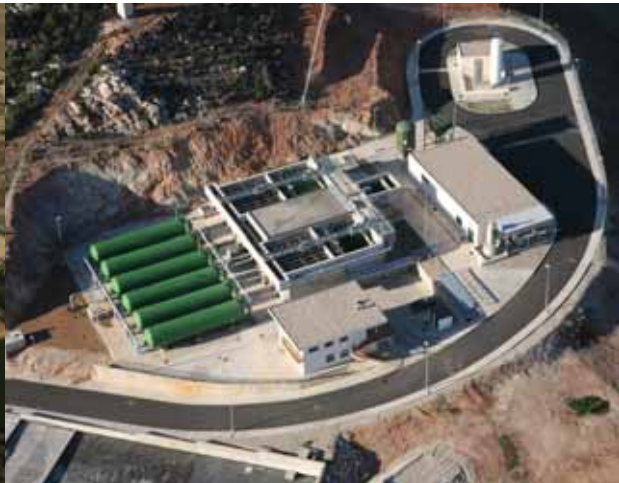
3. Design and construction supervision of the Puertollano water supply system
