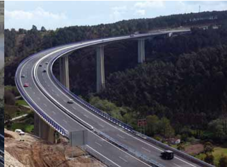
Widening of Viaduct of San Pedro de la Ribera
