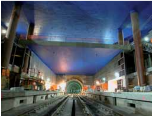
1. Construction supervision of the Madrid Metro. Line 12 expansion
