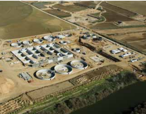
2. Construction supervision of the Estivel wastewater treatment plant
