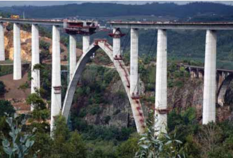
Viaduct of the Ulla river
