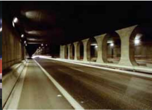
3. Construction supervision of the Bacerlona Ring Road Section: Vila Olimpica
