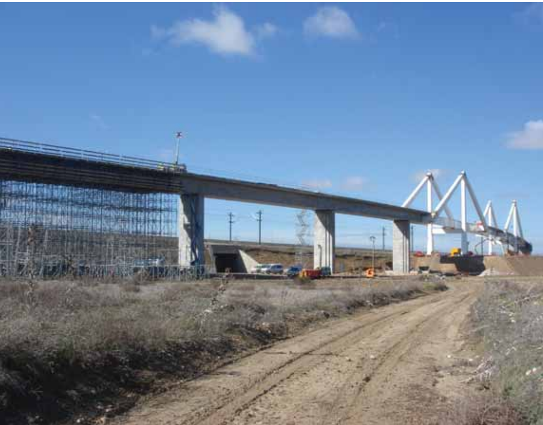
1. Construction supervision of the high speed railway from Valencia to Seville
