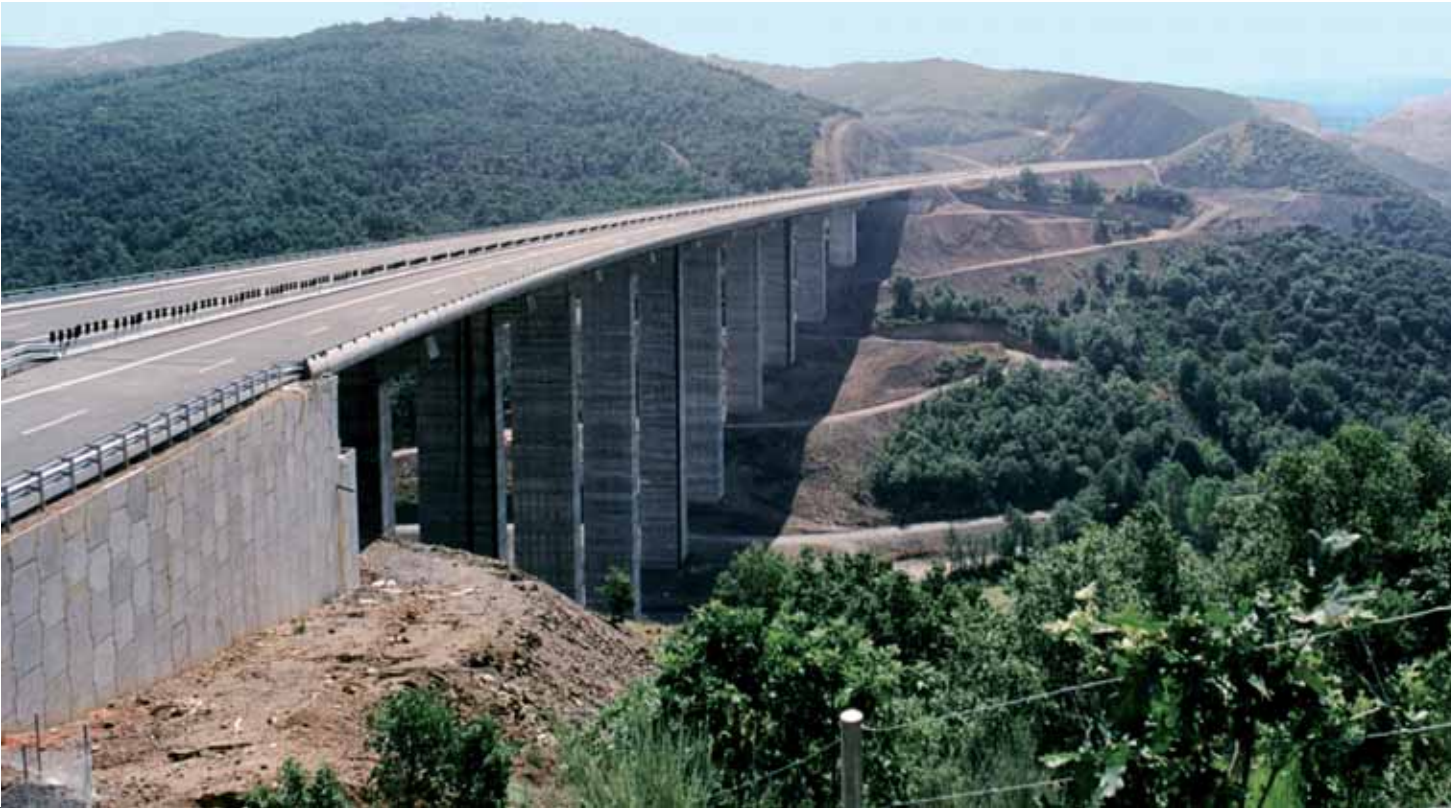
1. Construction supervision of the Bembibre bridge on A-6 motorway
