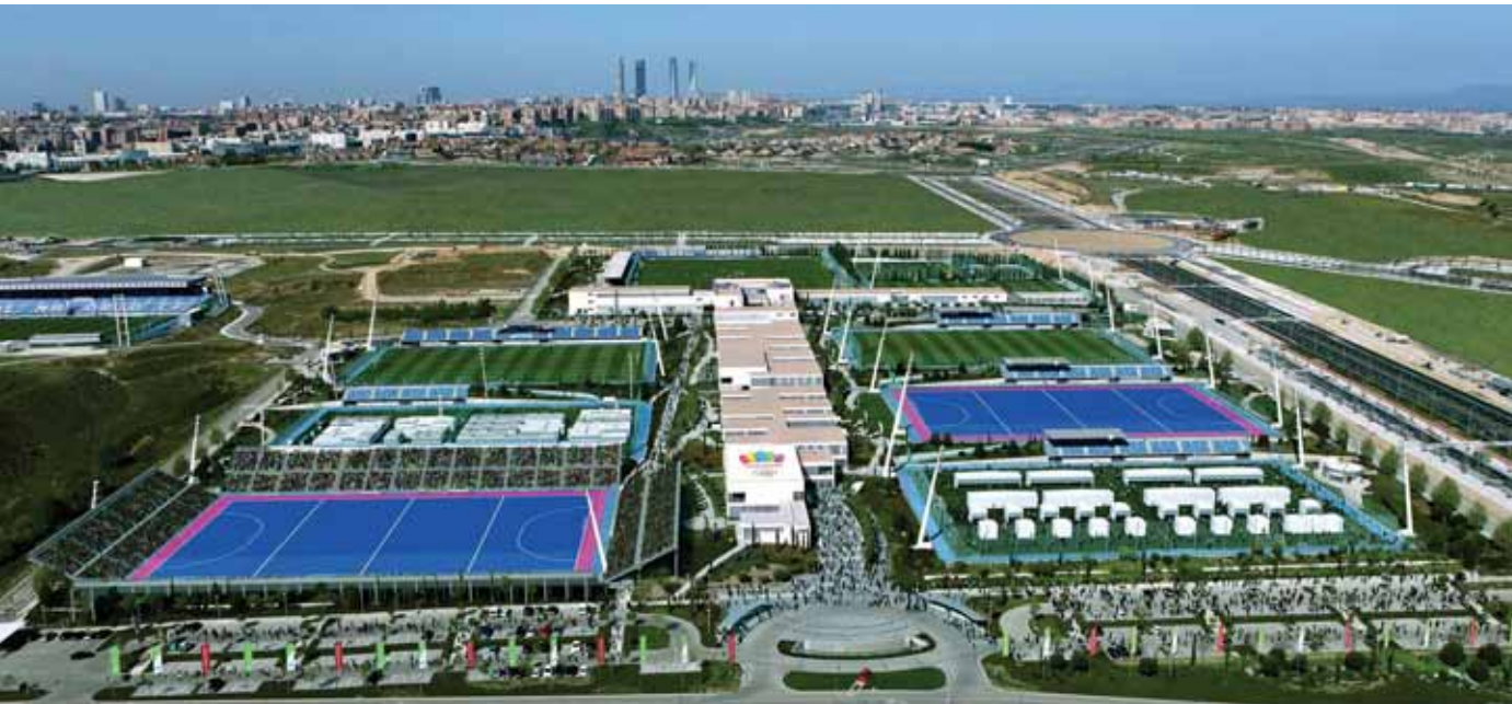
1. Madrid - SPAIN Design of the hockey venue at the Real Madrid Sports City
