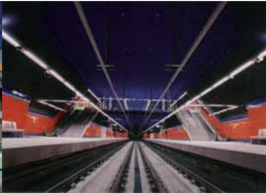
2. Construction supervision of the Madrid Metro. Congosto station on Line 1
